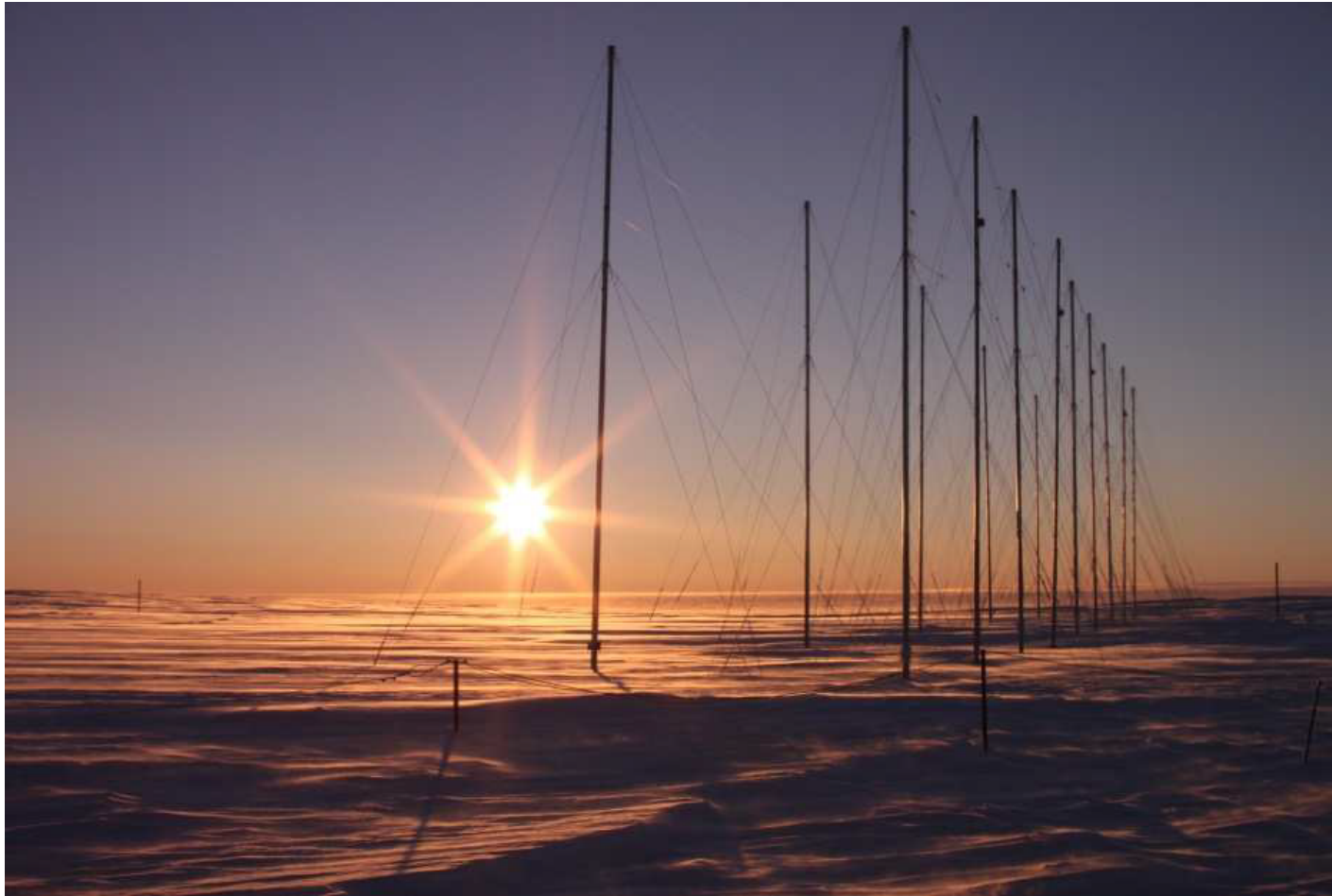
HF Antenna at SANA-E-4 Part of the SuperDARN radar network
