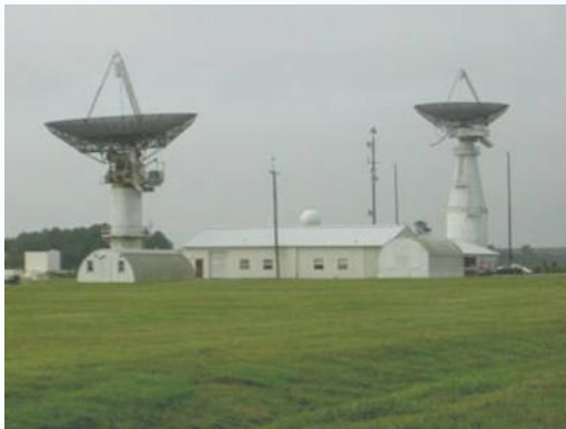
Wallops UHF on left, S-Band on right
