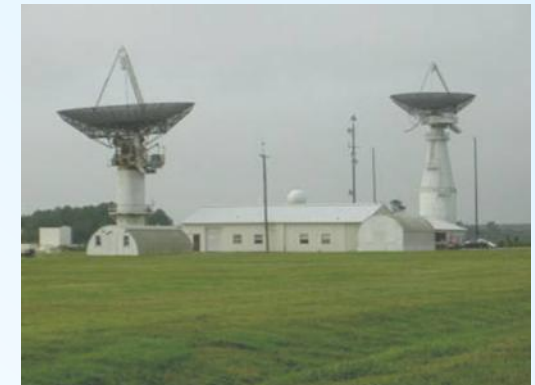
Wallops UHF on left, S-Band on right
