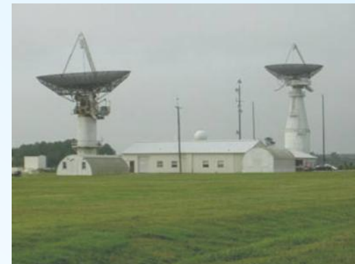
Wallops UHF on left, S-Band on right
