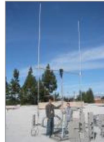
UHF Earth Station Construction
