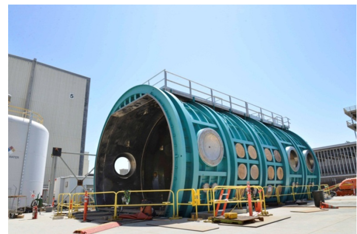
New TVC Under Construction
